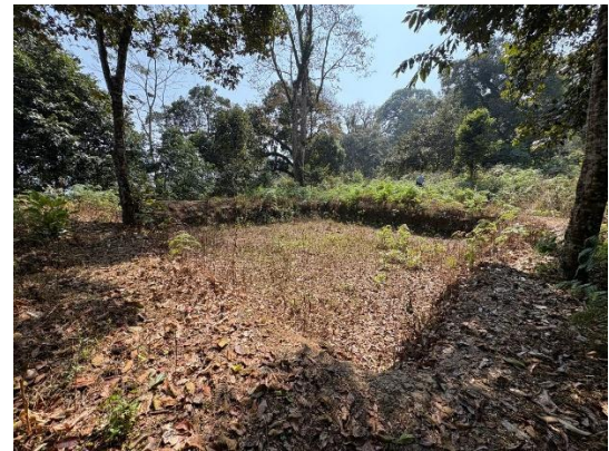
Figure 9: Catchment dug pit for water percolation at recharge zone
